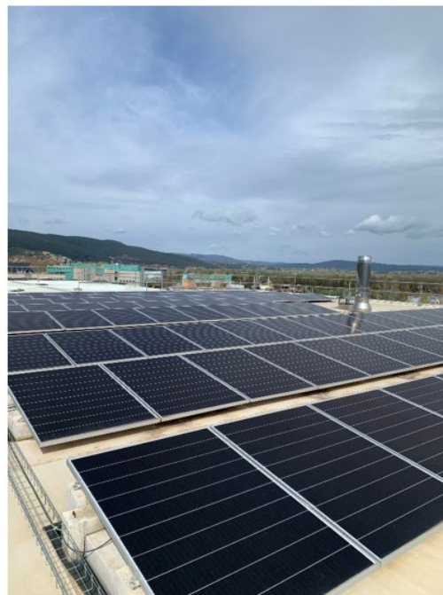
Figure15 - On the left 40 KW photovoltaic system; on the right 70 KW photovoltaic system.
