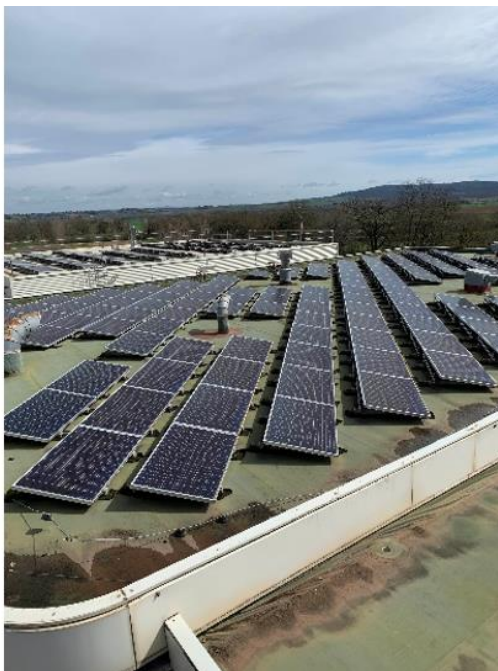
Figure 20 - On the left photovoltaic system 40 KW; on the right photovoltaic system 70 KW
